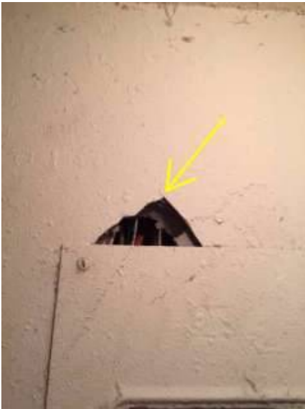
Photo 6-1 Opening in wall top of service panel.
