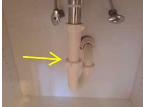
Photo X-2 Guest bath sink trap/drain in working order.
