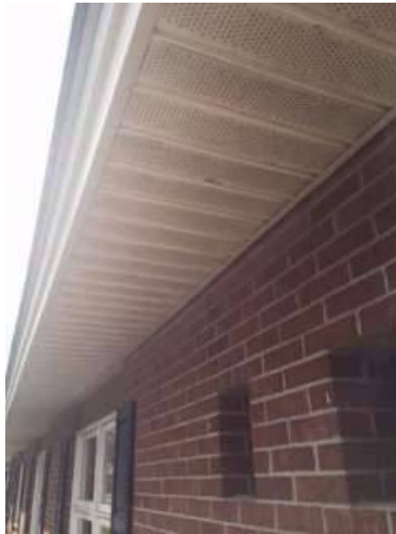
Photo X-34 Soffit vents in good standing condition.
