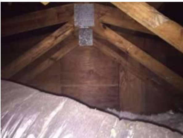
Photo X-3 View of attic.
