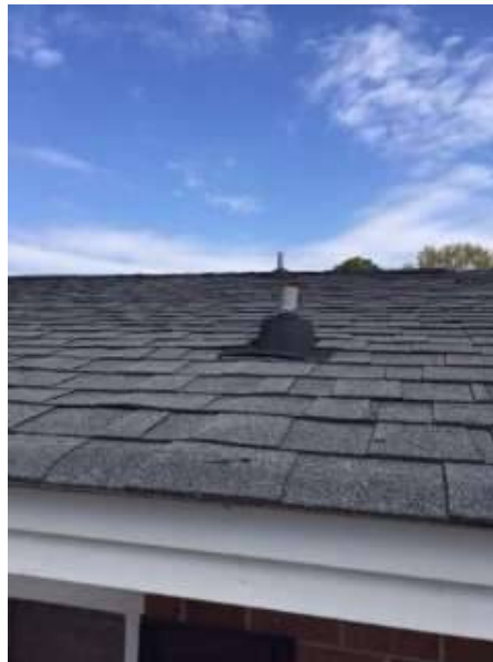
Photo X-16 View of Roof - In working order and serviceable.
