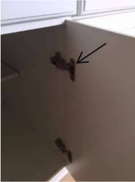
Photo 16-1 Hinge Adjustment in Kitchen.
