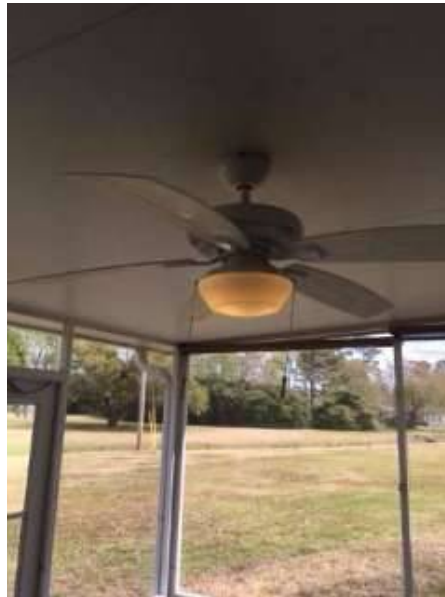
Photo X-22 Ceiling fan and light in screened porch in working order.
