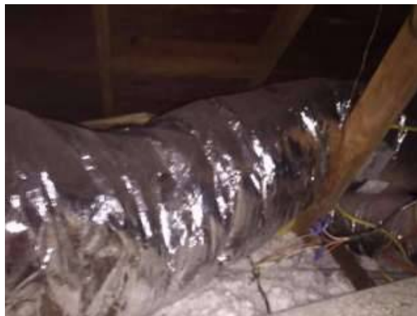
Photo X-4 View of attic duct work.
