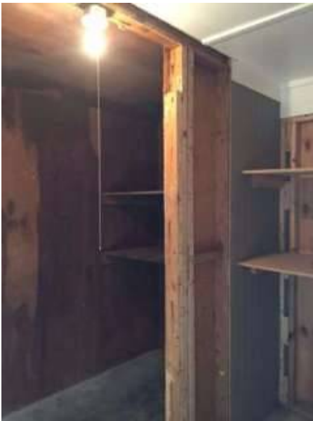
Photo X-31 Room at rear of Carport - Sound condition.
