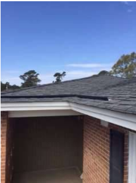
Photo X-15 View of Roof - In working order and serviceable.
