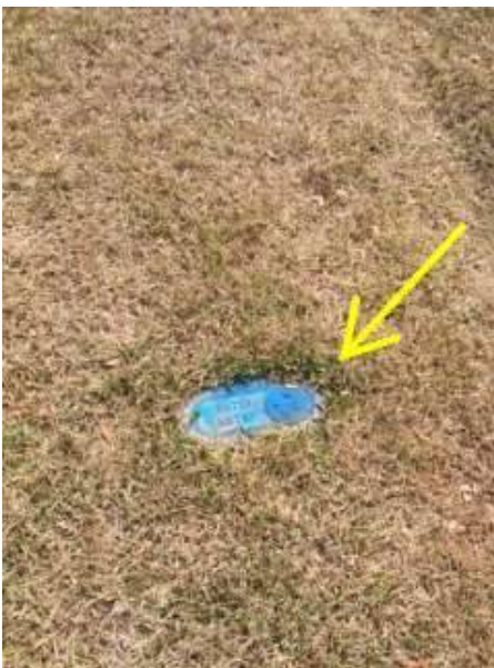
Photo X-11 Water shut off in front of property.
