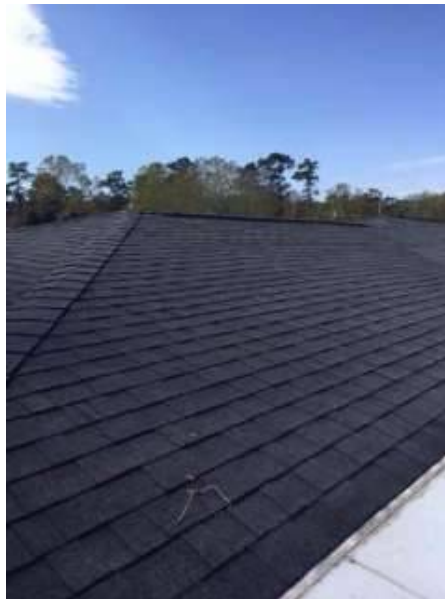
Photo X-20 View of Roof - In working order and serviceable.
